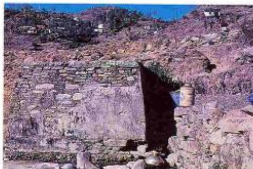
Plate 1. A tank constructed to conserve spring water
