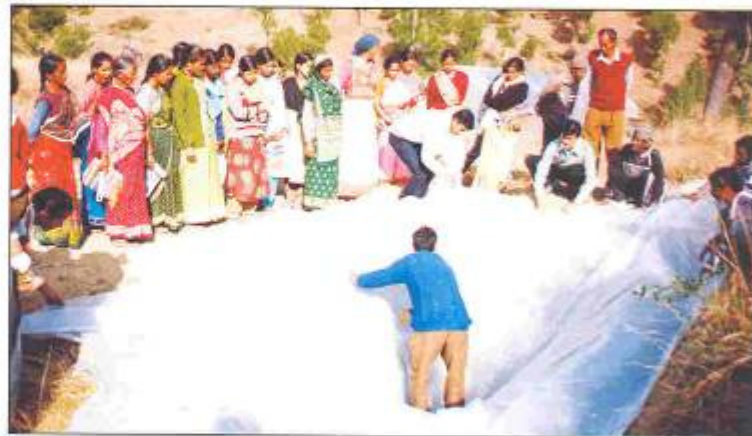
Fig. 60. Demonstration of poly-pond construction in Railakot village
