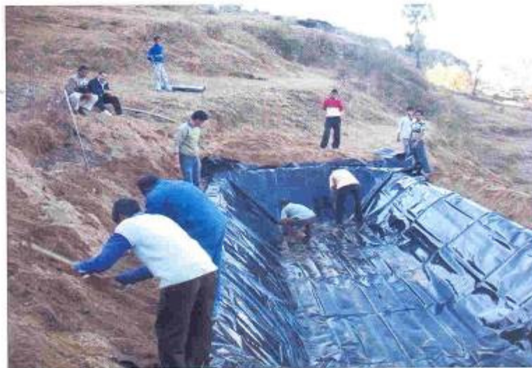
Fig. 38. Construction of waterharvesting tank
