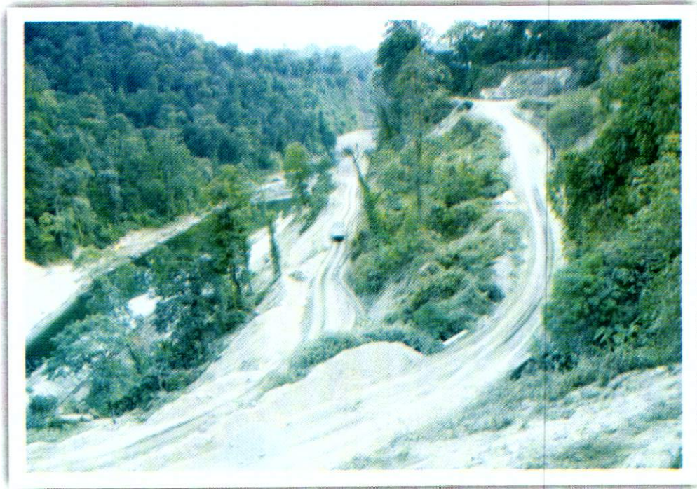
Fig.37. A fragmented flow view in the downslope of Rangnadi HEP (405 MW) in Arunachal Pradesh.
