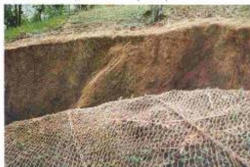
Fig. 2. Bio-engineering stabilisation with jute/coir netting as a surface protection measure being used in a landslide affected site in Mamlay watershed
