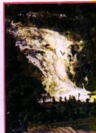
Fig. 25: Mile 9 landslide on NH31A.
