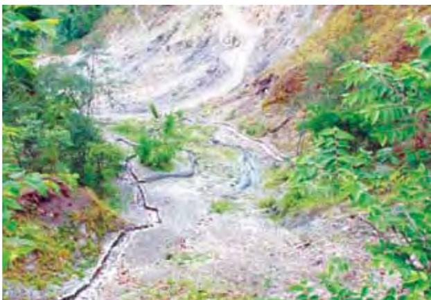
Fig.6. (a) Engineering measures (catch water drains) in Bojeck landslide
