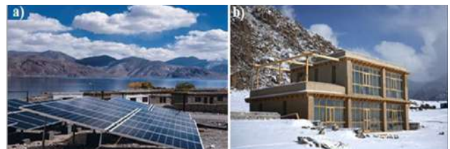
Fig.3: (a) Solar Panels installed at Pangong (b): Passive Solar House
